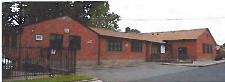
Existing community center at Alder Grove
