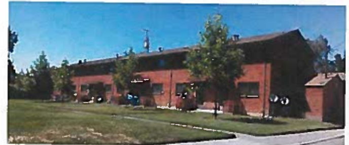
Existing Alder Grove Public Housing
