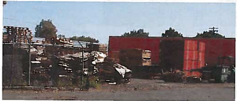
Industrial area east of 5th Street looking eastward. Area is characterized by no sidewalk, chain link fences, industrial storage yards, and lack of landscaping. Although this is a legal use in the M-1 zone and consistent with pre-existing code, this site does not meet current planning and development standards for the M-1 zone.
