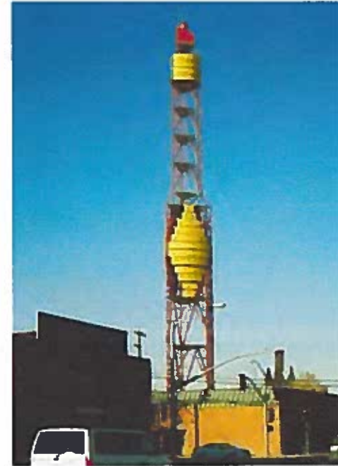
Iconic 300-foot tall weather tower at KXTV broadcast facility
