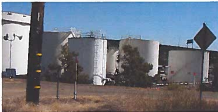
View of the Tank Farm from Broadway
