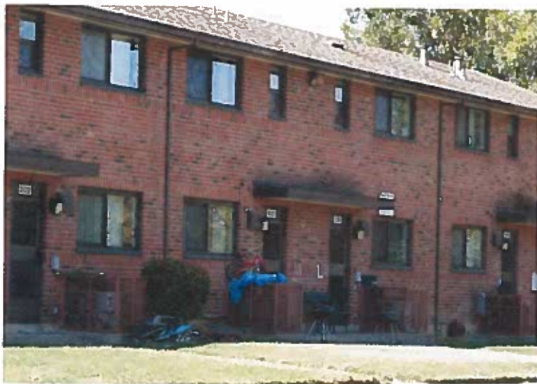
Existing building at Alder Grove
